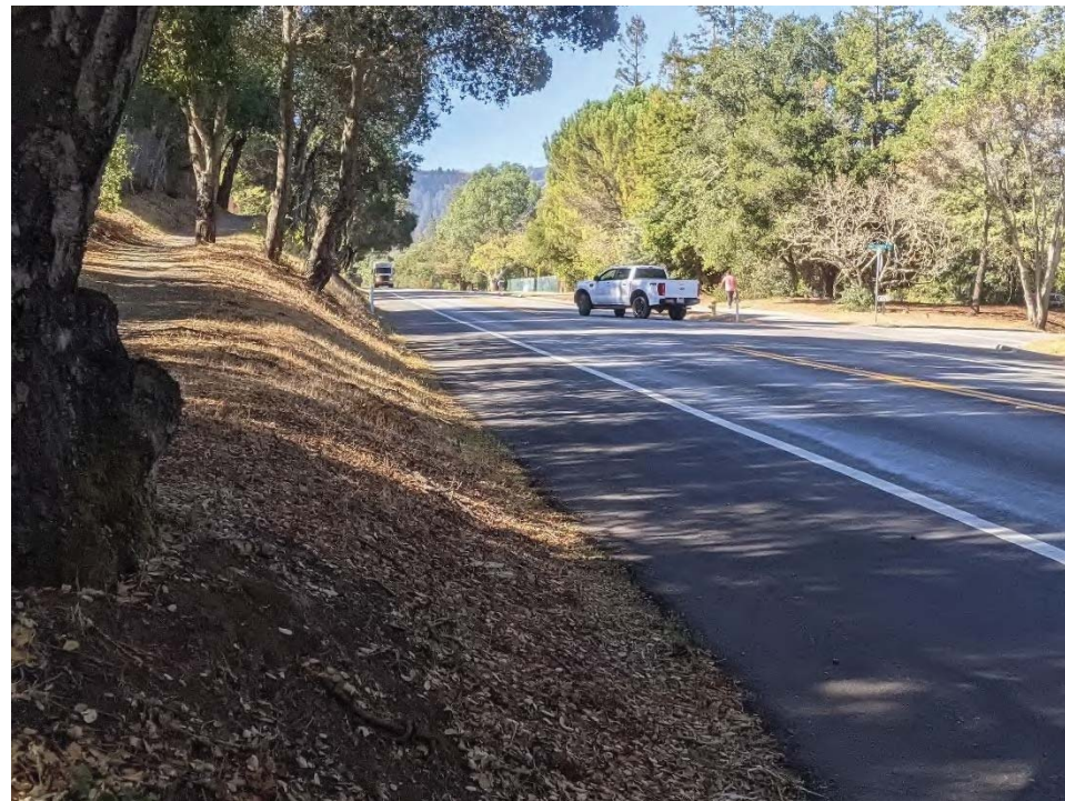
Original Alpine Rd Driveway Looking West
