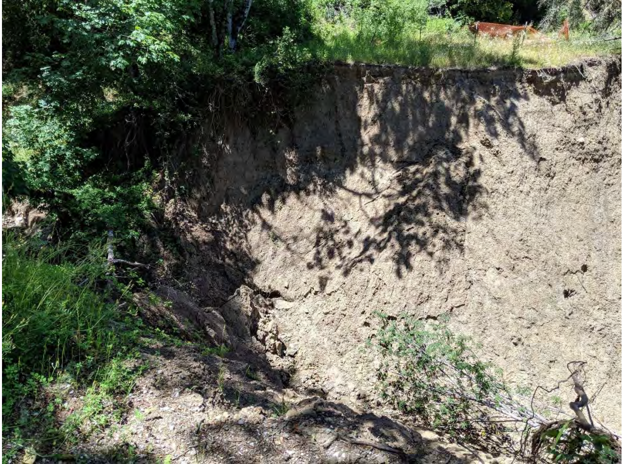
Photo 4. Delineated other Waters at Data Point P01, showing incised, failed slope in eastern portion of study area corridor.
