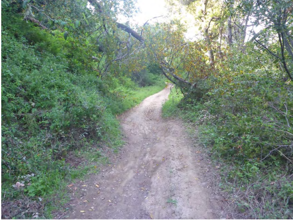
Photo 5. Representative photograph of access road within study area, showing minor rills from sheet flow after heavy rains.
